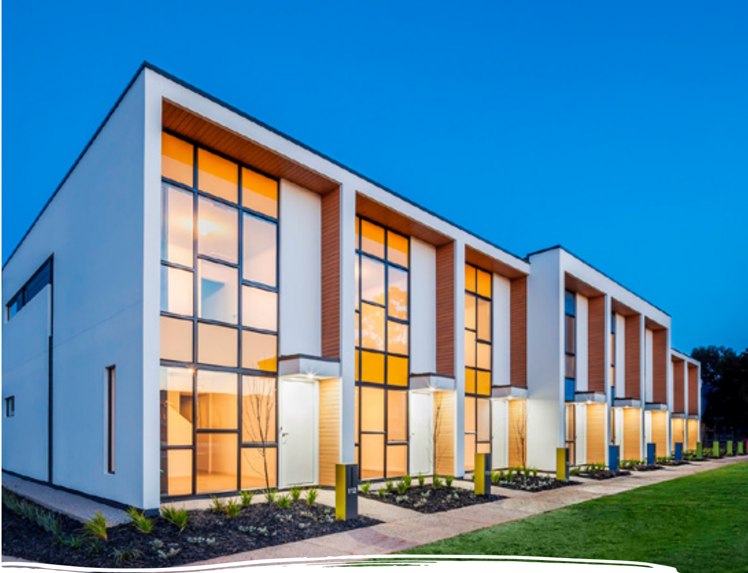
Unity Housing, SA - St. Clair affordable rental housing project
